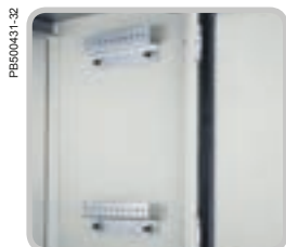
Perforated rails installed on lateral studs.
